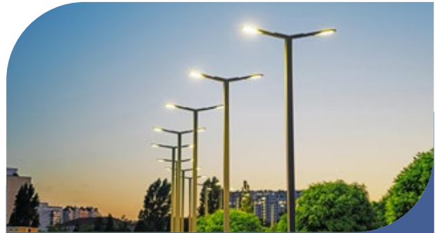
LED lighting for streets, common areas in projects, and etc, to reduce energy consumption throughout project lifecycle.
